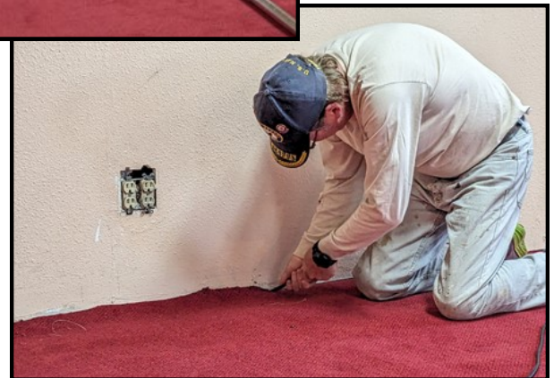
BELOW: Rock Slaughter works at tucking the edges of the carpet.
