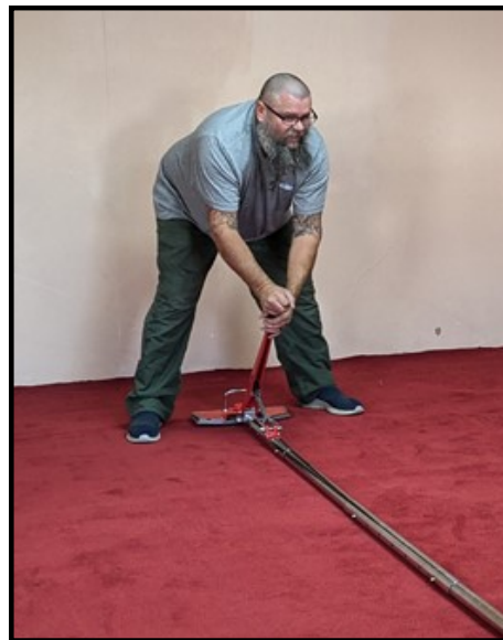
LEFT: Brent Heath puts the stretch on the new carpet.
