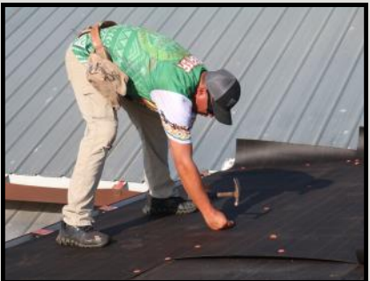
Ronald Rolin and Duck Weaver, left, along with Randall Ward, right, work to replace roll roofing on a portion of Grace Point Ministry Center.
