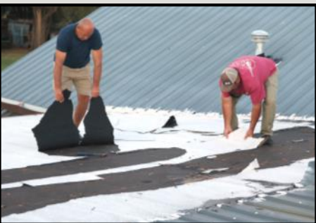
Ronald Rolin and Duck Weaver, left, along with Randall Ward, right, work to replace roll roofing on a portion of Grace Point Ministry Center.
